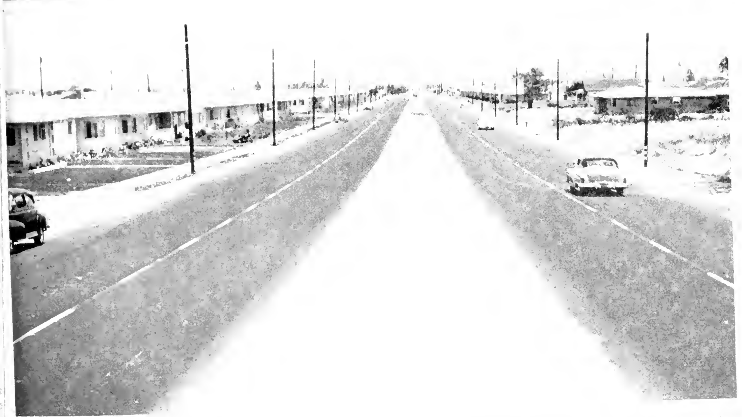
UPPER: Looking westerly from Inglewood Avenue showing completed divided highway development along Redondo Beach Boulevard. LOWER: Looking easterly from Hawthorne Boulevard along completed 4-lane divided highway development on 174th Street.
